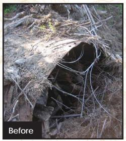
Before it was replaced, debris would regularly clog this undersized culvert.
