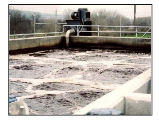
In suspended-growth systems, the sewage is mixed by aeration within an aeration basin, or in a treatment tank in the case of a residential scale system. This produces a mixture of water, microbes, and sewage known as activated sludge.
