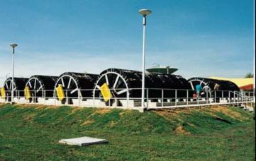
Aerobic treatment units, also known as aerated tanks or extended treatment plants, utilize an aerobic (oxygen rich) process, and remove substantial amounts of BOD<sub>5</sub> and TSS not removed by primary treatment.
