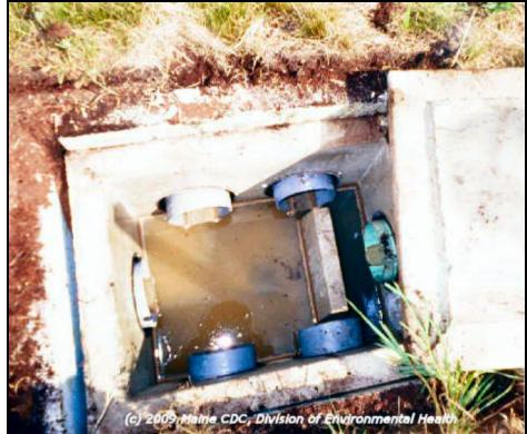
When septic tank additives are used, instead of remaining in the tank, the liquefied fats, grease, and solids leave in the effluent and enter the field. Much of this material is not subject to bacterial breakdown in the absence of oxygen, can significantly shorten the life of the field by reducing soil permeability.
