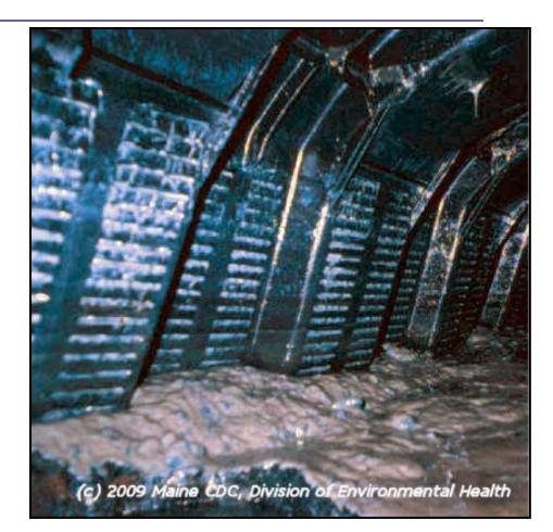
Once the biomat is established, the organisms in the mat are extremely effective in stabilizing organic waste, removing particulates, and removing pathogenic organisms. Bacterial indicators of pathogenic contamination are total coliforms, fecal coliforms, and fecal streptococci.
