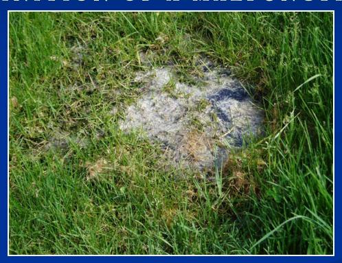
Ponding or outbreak of wastewater or septic tank effluent onto the surface of the ground.
