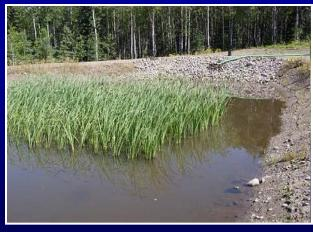
In 1993 the Chewonki Foundation received approval for a constructed wetland system. The system used the lower portion of a concrete septic tank, and cattails as the vegetation.
