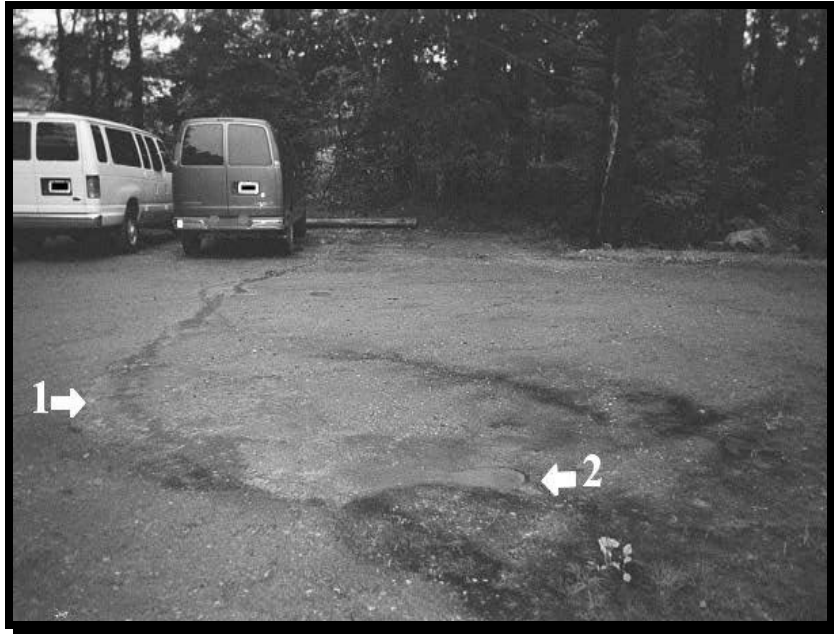
Fig. 3 Malfunction resulting in effluent runoff (1) and breakout (2).
