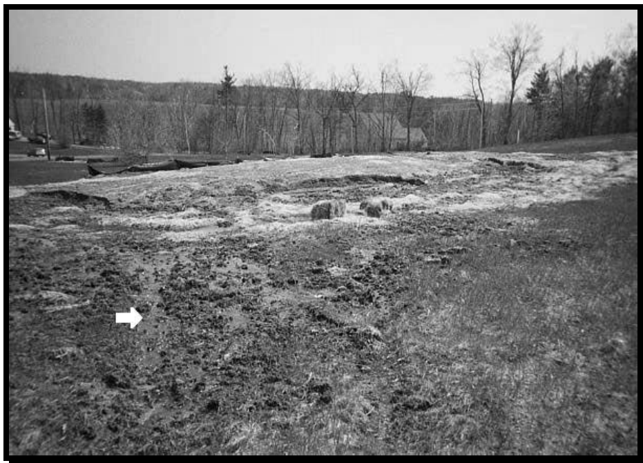
Fig. 2 Malfunction resulting in effluent breakout and ponding (arrow).
