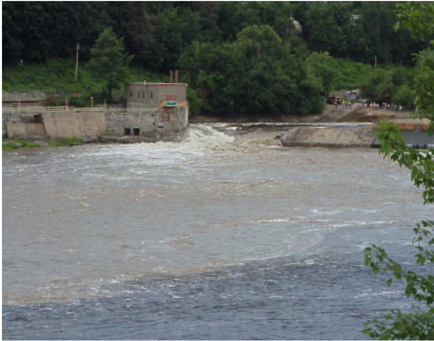
Breaching of the Edwards Dam, July 1, 1999
