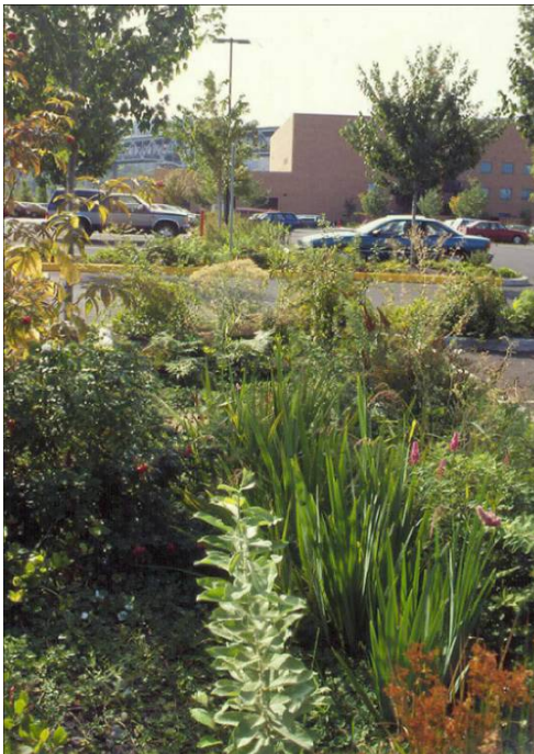
Figure 1: Vegetated Filter Strip
