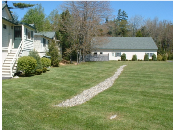
Figure 6.4 - Photo of Infiltration Trench
