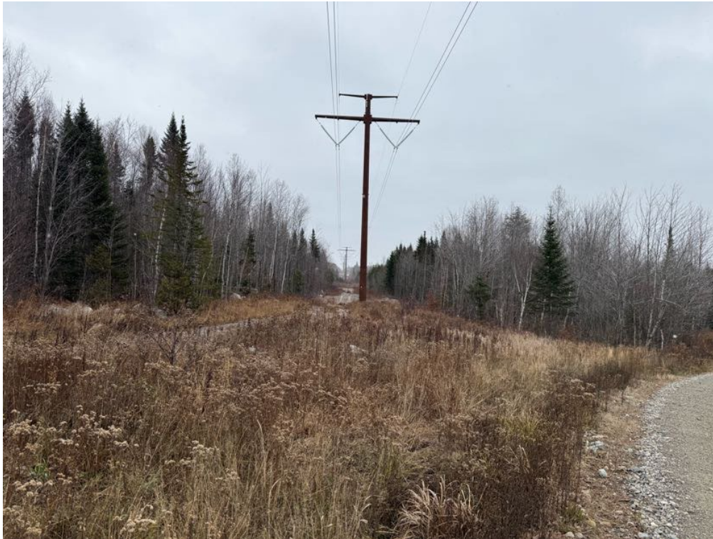
Site 3 (Looking East and West, respectively):
