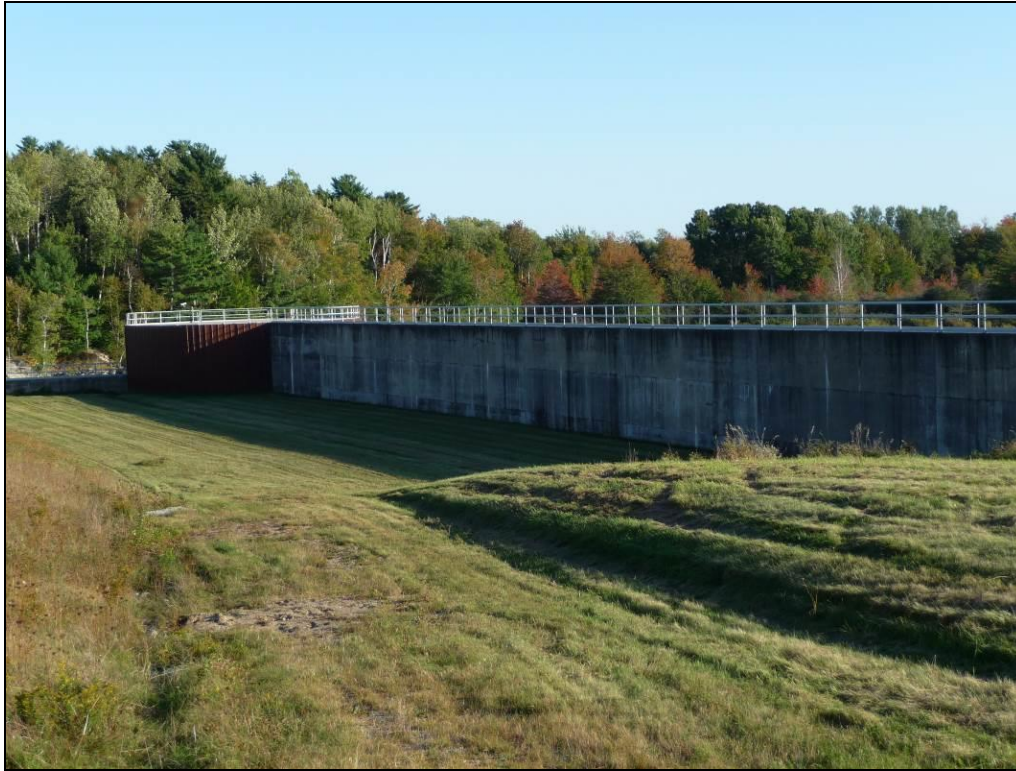
Photo A-5: Graham Lake Dam Flood Control Structure
