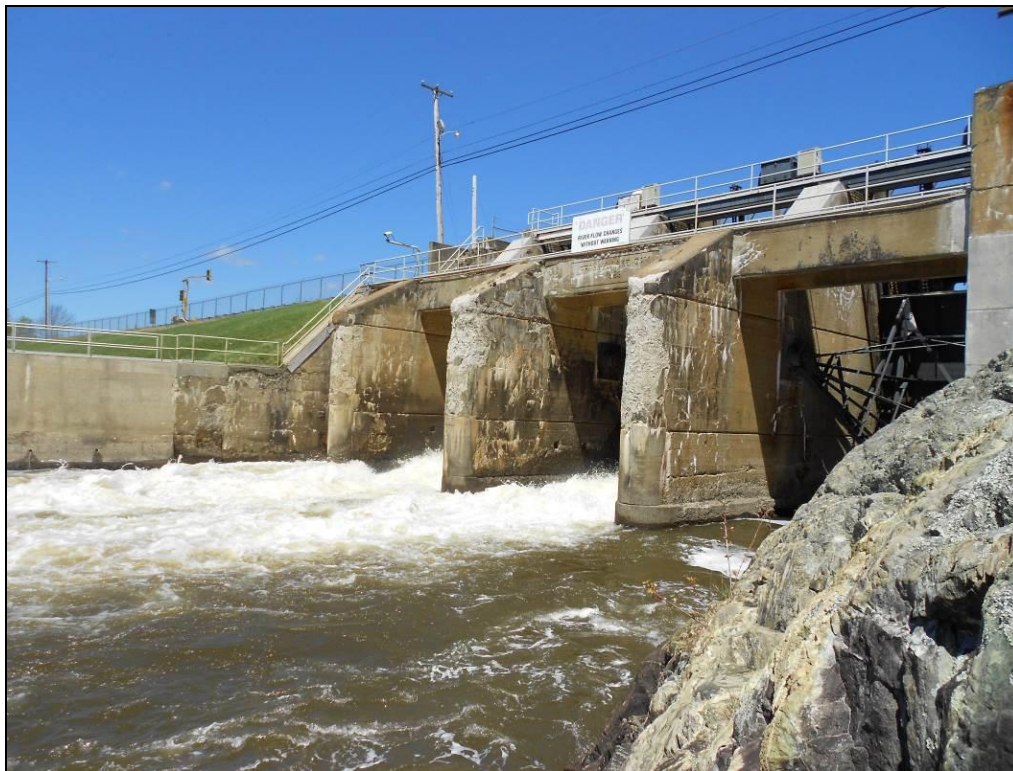
Photo A-4: Graham Lake Dam Gate Structure
