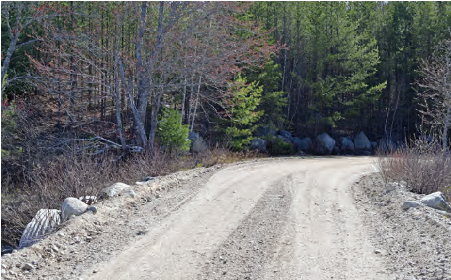
P19 - View looking west on Shadagee Road over Mopang Stream in T24 MD BPP. This location is used as an unofficial water access point for Mopang Stream.
