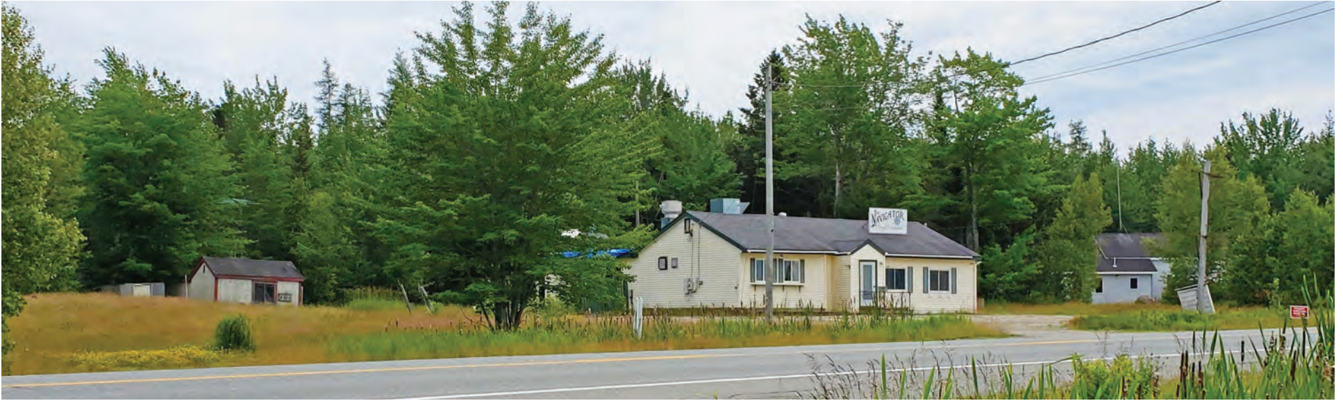
P68 - View looking southeast towards the site of the proposed O&M building off Route 1 in Columbia. The existing building will be replaced with new construction. The building will be visually compatible with the surrounding commercial buildings.
