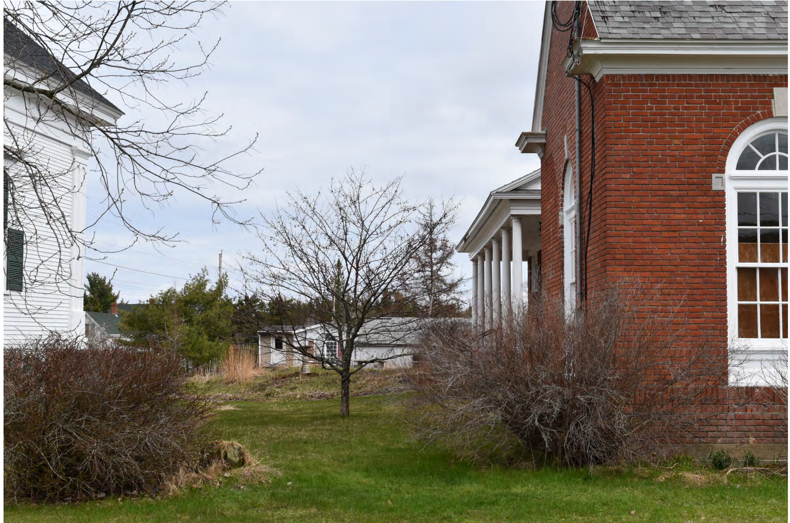
Gallison Memorial Library front of library Normal View Existing Conditions
