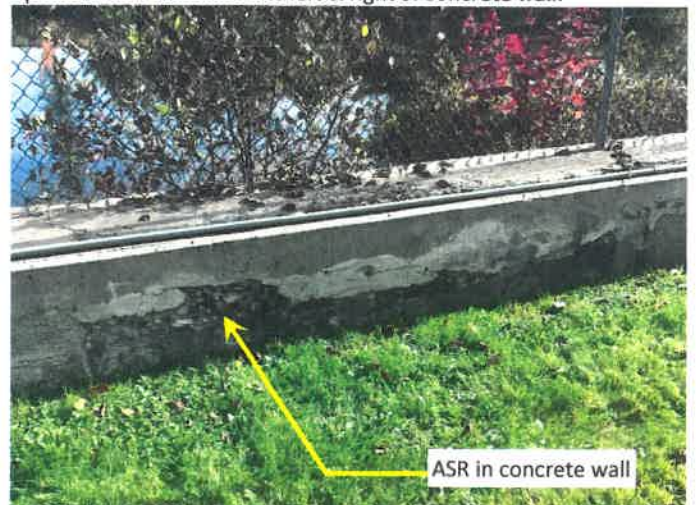
4. Concrete wall between left abutment & bridge.
