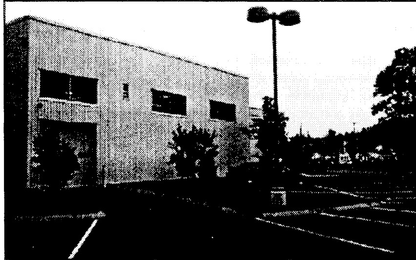
An Exterior Light Designed to Shine Down and not Light the Night Sky
