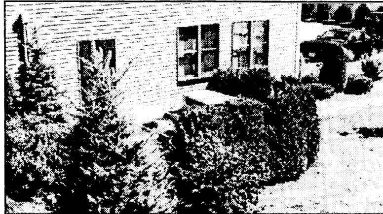
Exterior Air Conditioning Equipment Shielded by Landscaping
