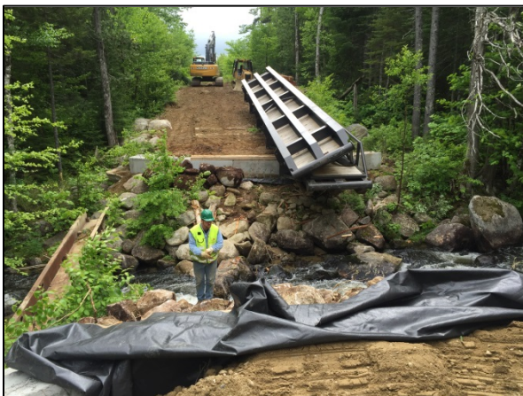
Installation of a management road bridge in the Eastern Region
