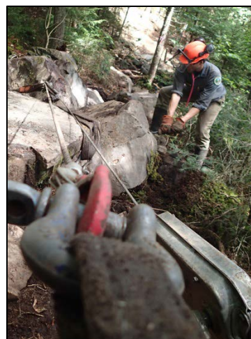
Trail construction in progress in the BPL Western Region.
