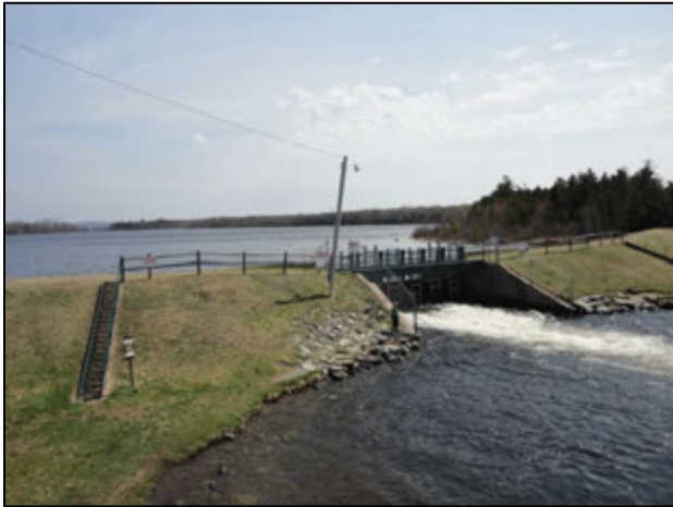
West Outlet dam.
