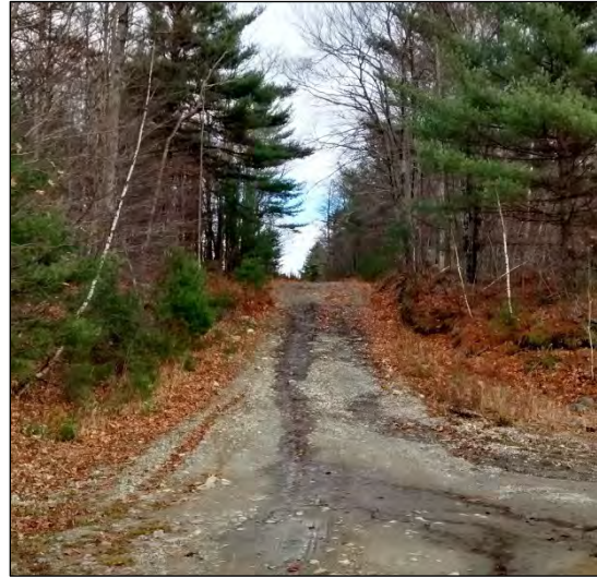
Eroded slope on Vienna Mtn Road (prior to recent BPL work)
