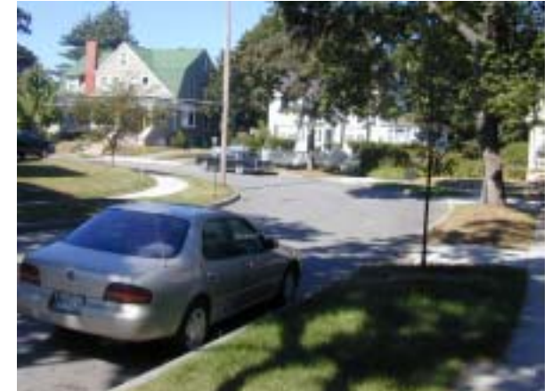
A 24’ wide road allows room for on street parking and a channel for through traffic.
