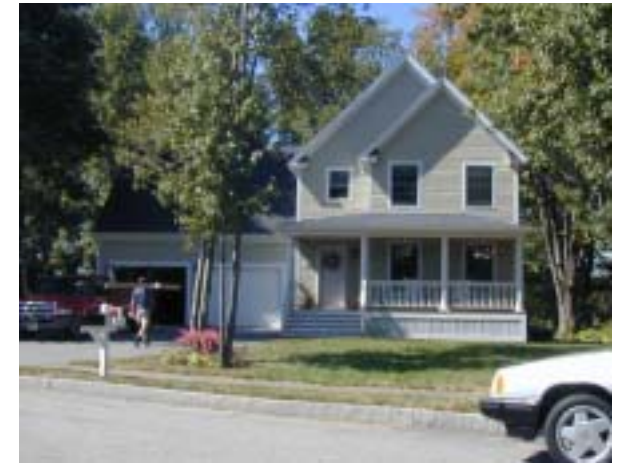
Twin gables and porch face the street while broad steps emphasize the location of the front door.
