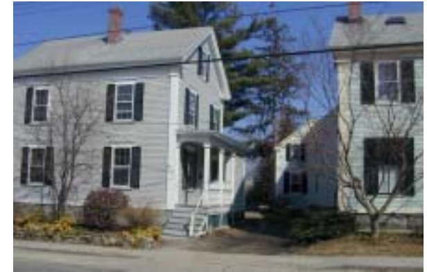
If the gable ends of these houses faced the street the side yards would have been larger and more private.
