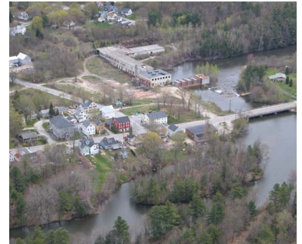
An example of an infill site: an abandoned mill surrounded by established neighborhoods and commercial areas.
