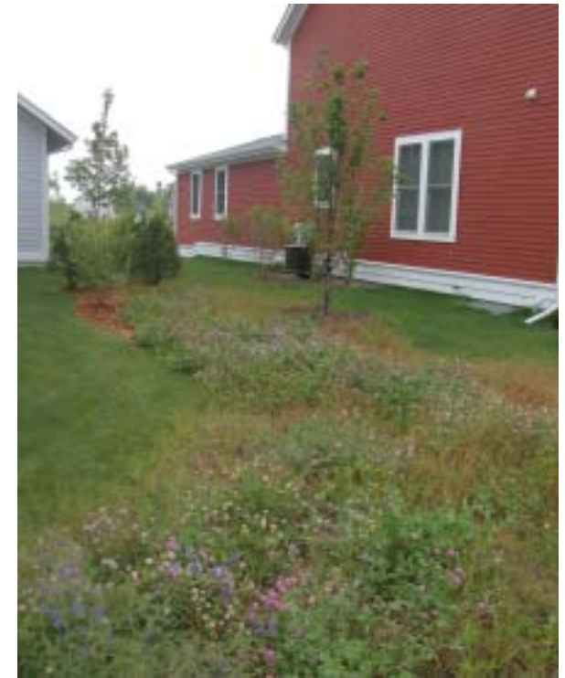
This side yard is a functional part of the stormwater system, using native grasses and wildflowers to help purify runoff in a shallow drainage swale.
