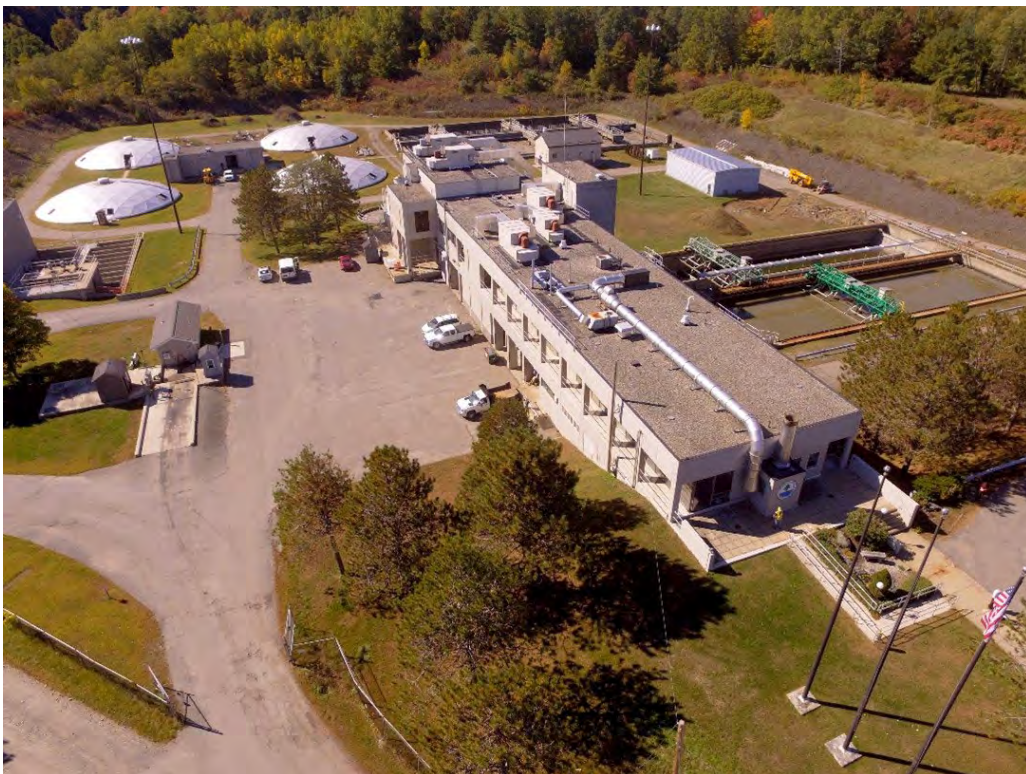
1- Aerial Photo of Kennebec Sanitary Treatment District Treatment Plant at 401 Water Street.
