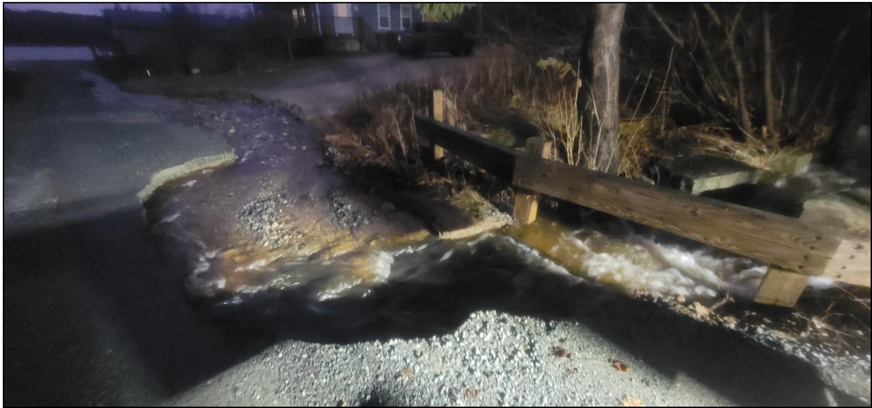
Figure I-3: Sullivan Culvert, 2023/2024 Storm Damage
