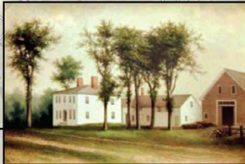
The Manning House Built 1804, N.R. 1993
