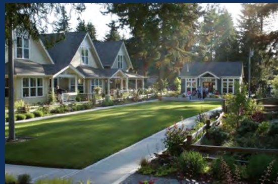
Cottage Court Development (where many smaller cottages face a central courtyard, with parking on the side, rear, or on-street)
