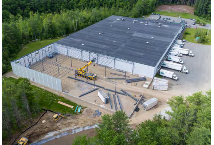
Expansion of Renys office and distribution center, located in Newcastle.
