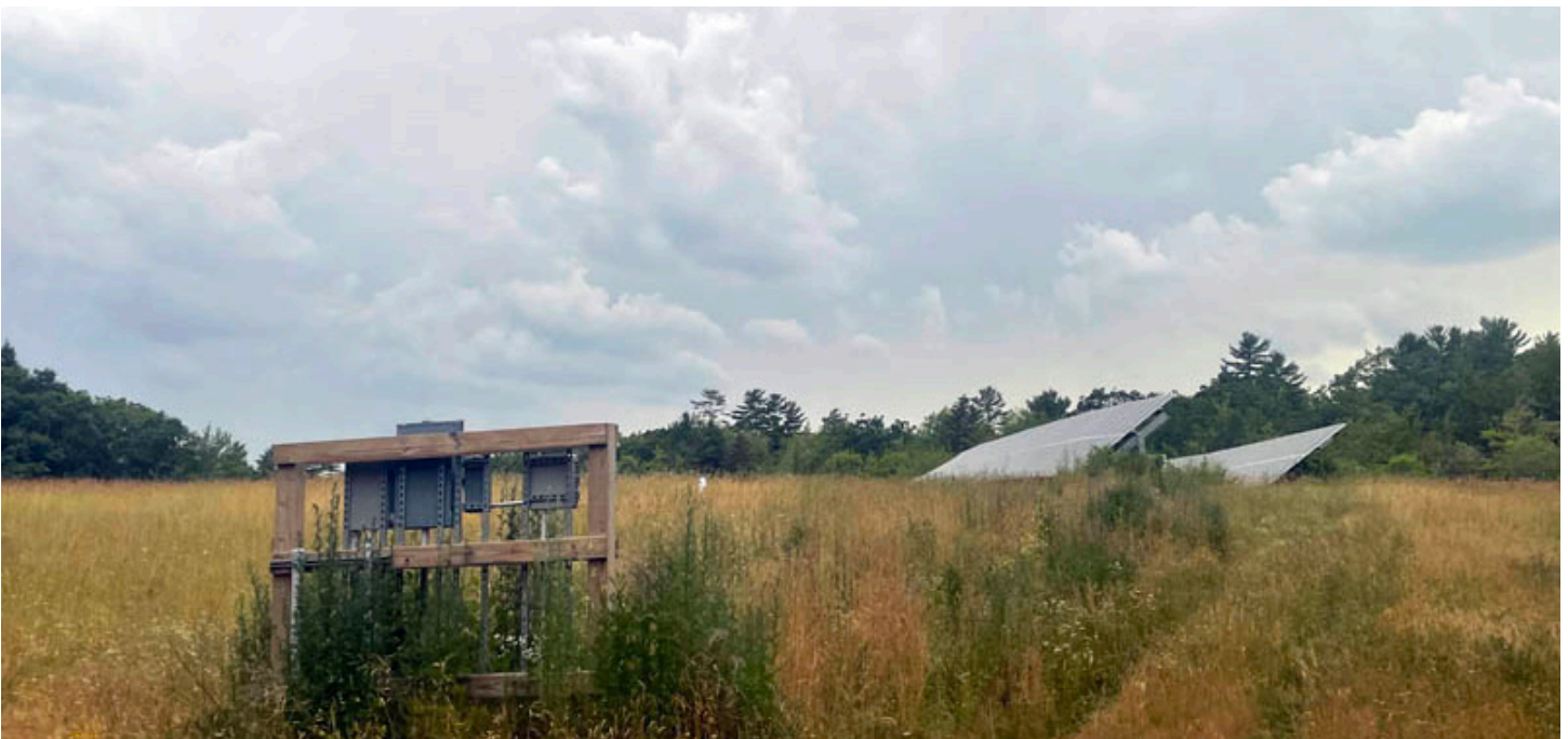
Damariscotta's town solar array
