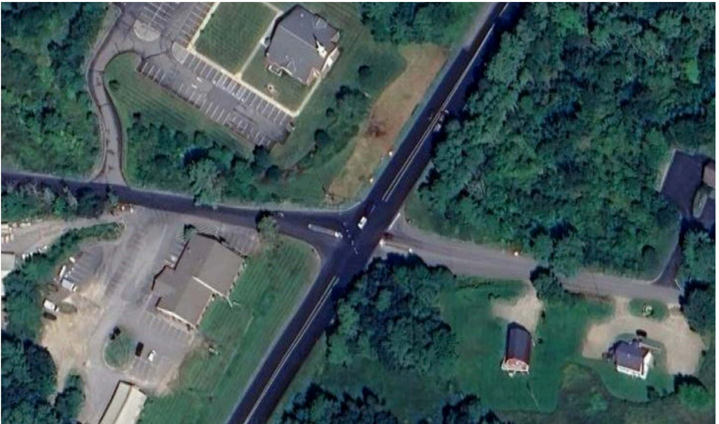
Intersection of Belvedere Road and Route 1
