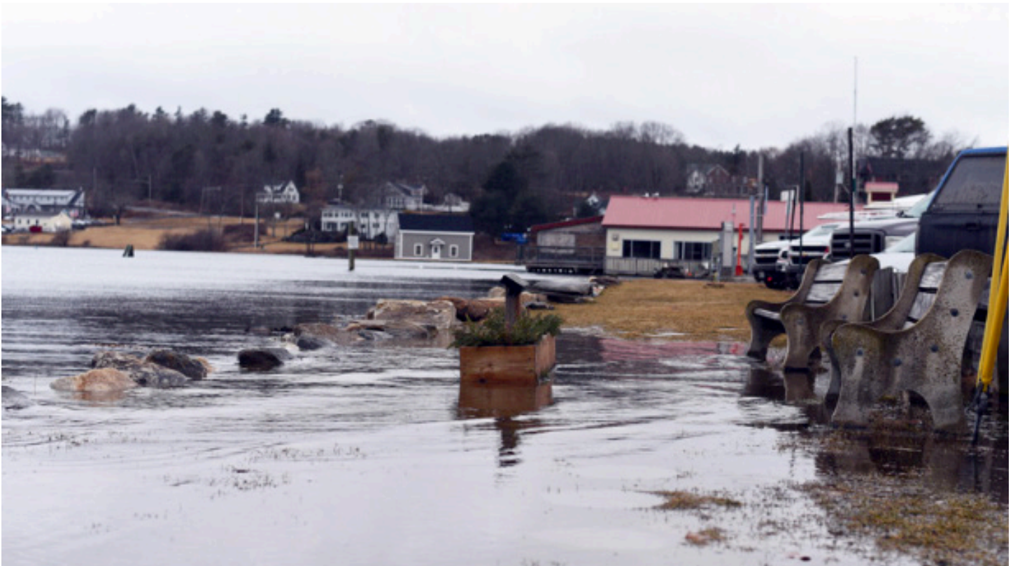
View of the flooded seating area adjacent to the downtown parking lot in 2018. Photo c/o Jessica Picard of the Lincoln County News.
