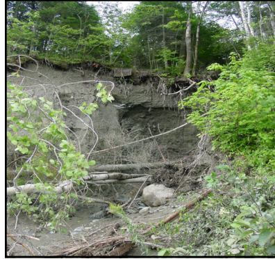
Riverbank erosion along the St. John River after heavy rains in 2004
