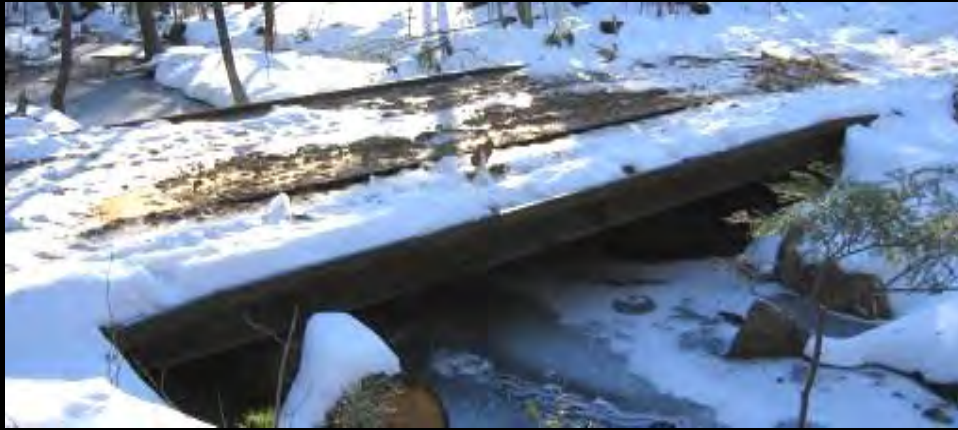
Temporary Bridge Deck
