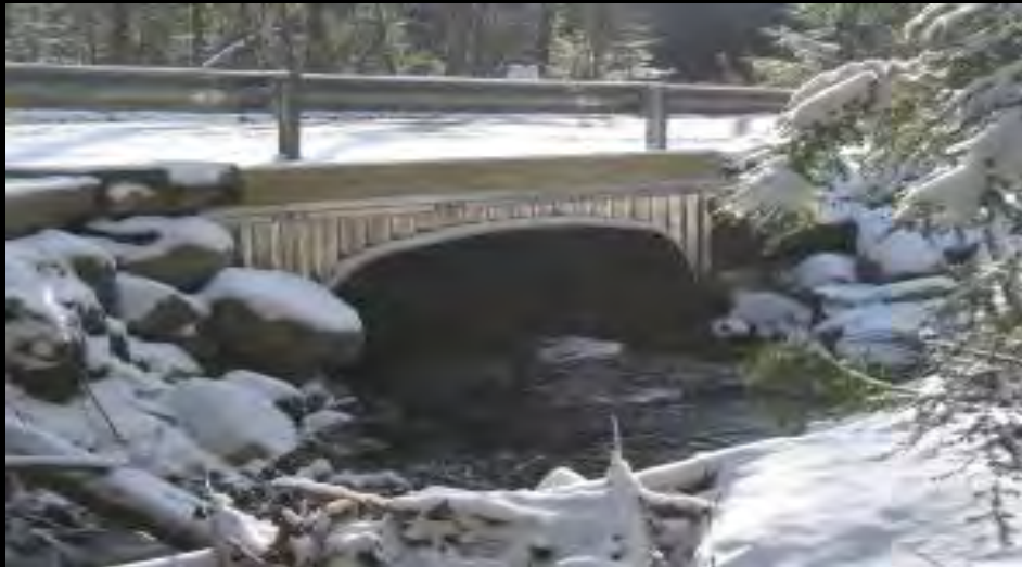
Bottomless Box Culvert
