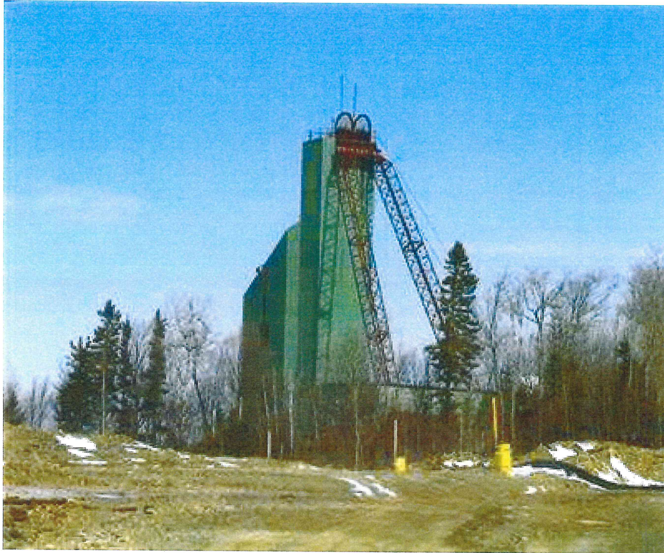
Headframe, Caribou Mine
