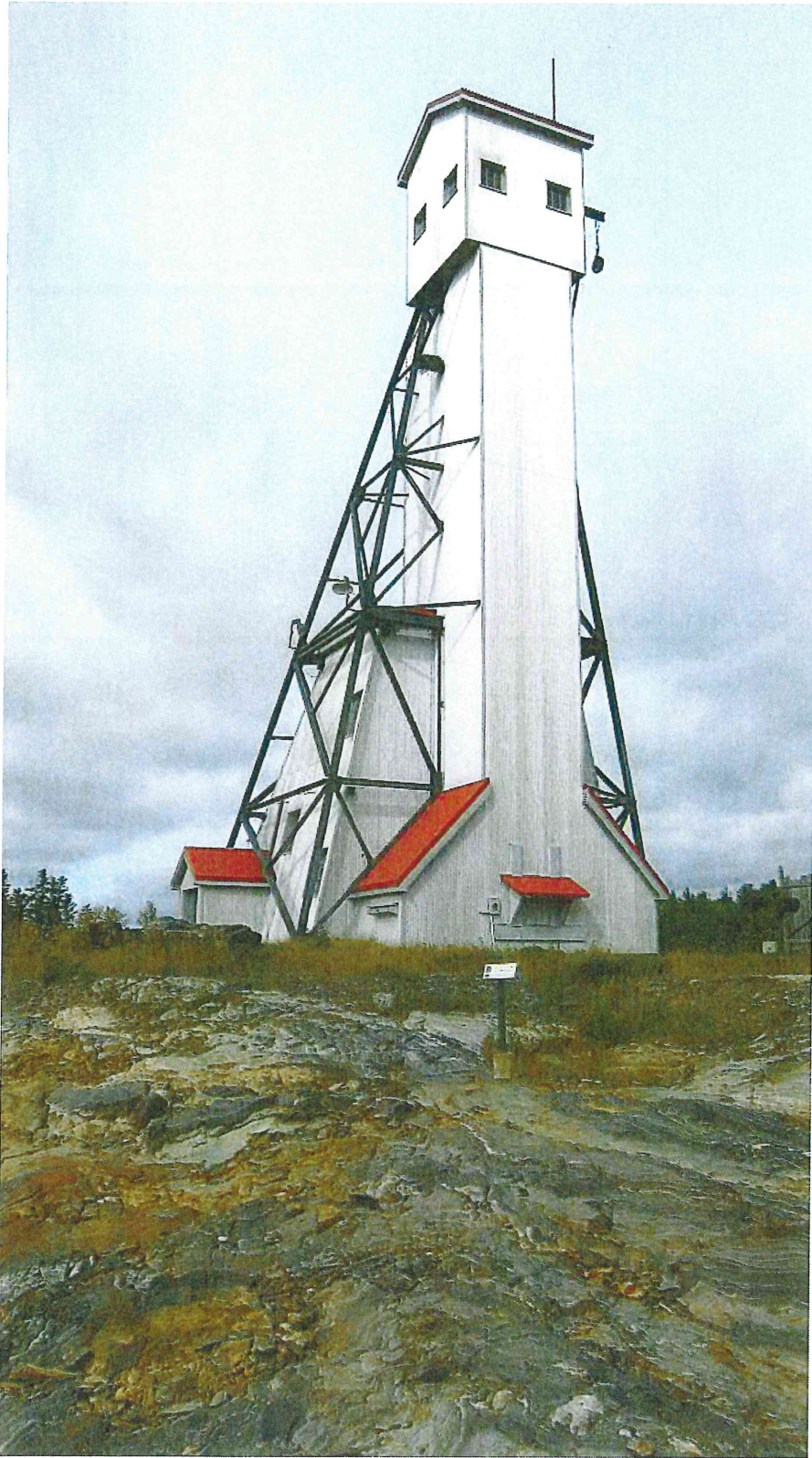
Headframe, Mcleod Cockshutt Mine
