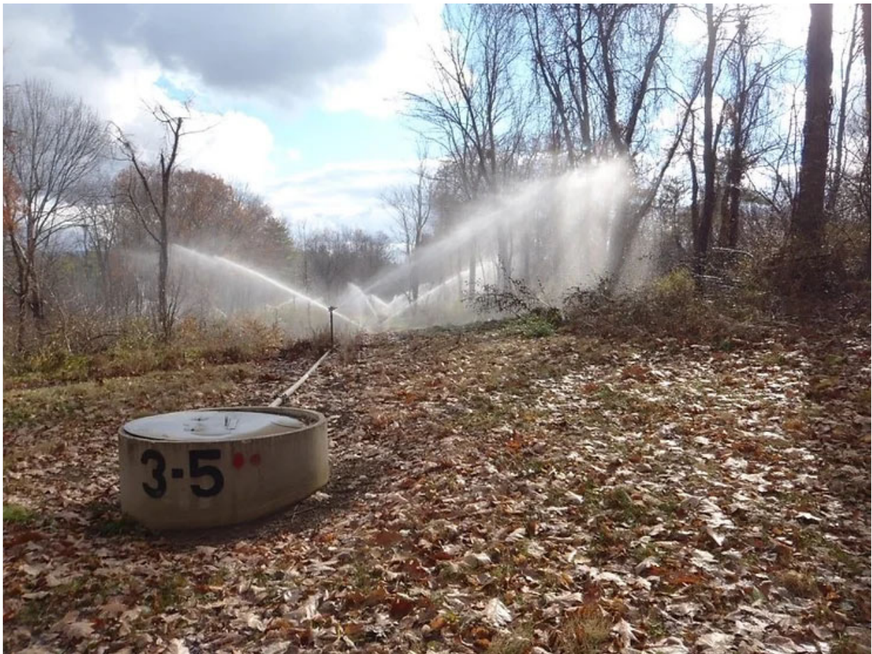
WASTEWATER SPRAY IRRIGATION SYSTEMS
