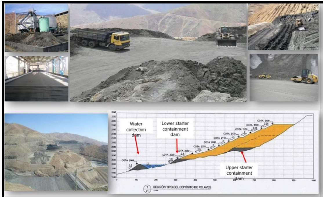
Figure 2-19 Cerro Lindo Moist Cake Disposal (1:2 Slope)
