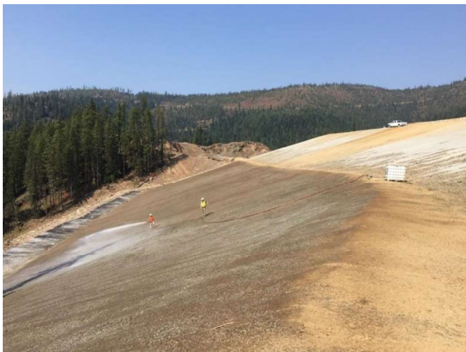
Figure 1 Spraying temporary sealant on a mine waste repository
