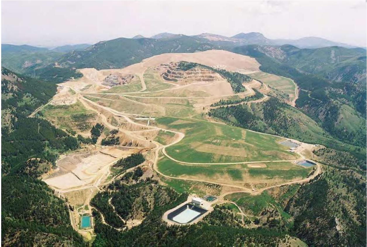
Landusky Water Treatment Plant, 2004. BLM Photo.
