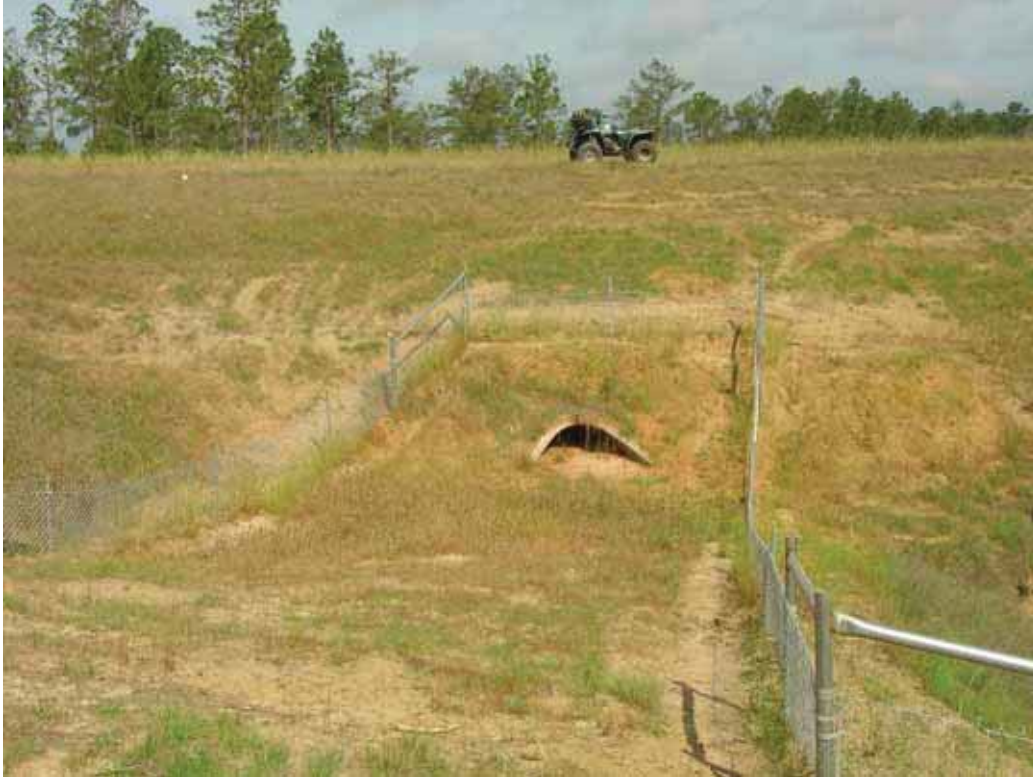
Figure 23. Photo. Fences lead gopher tortoises towards a culvert along Highway 63 in Green County, south of Leakesville, MS (copyright: Chuck Walters, Environmental Division, Mississippi Department of Transportation).
