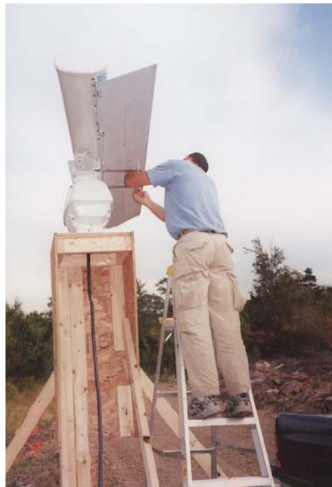
Photo 25. Angled bracket being installed on radar antenna.
