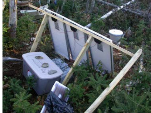
Photo 28. Acoustical monitoring stations on Black Nubble, with solar power array, batteries and instrumentation. Microphone is situated to far right in photograph.
