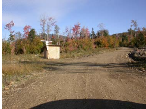
Photo 23. Black Nubble radar site.
