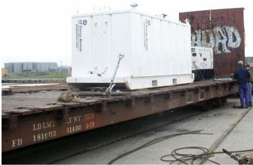
Diesel generator on train, as power supply to "turner gear device". (US "High Winds" Project)
