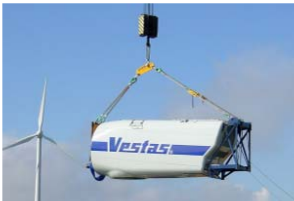
The unloaded nacelle lift adapter ready for return shipment - Total weight: 52000kg
