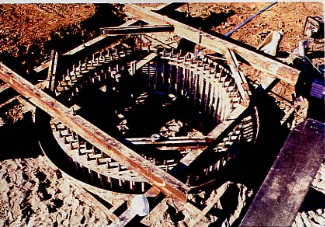
BACKFILLED INNER CMP WITH ELECTRICAL CONDUITS INSTALLED
