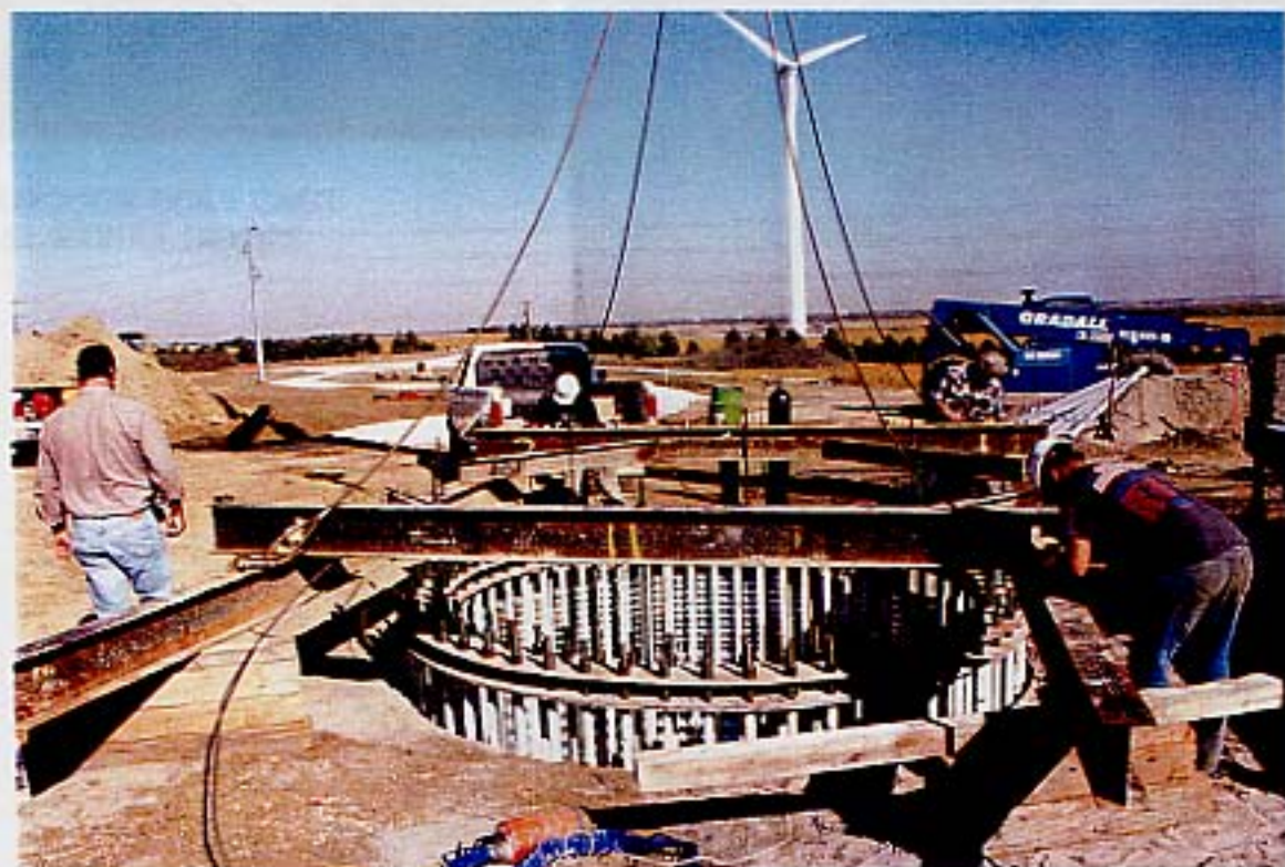
VIEW OF ANCHOR BOLTS LOADED INTO TEMPLATE
