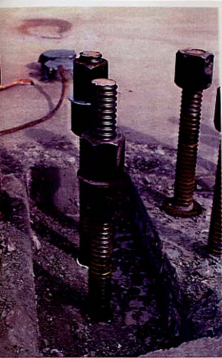
LEVEL BLOCKOUT VOID AFTER REMOVAL OF STYROFOAM
