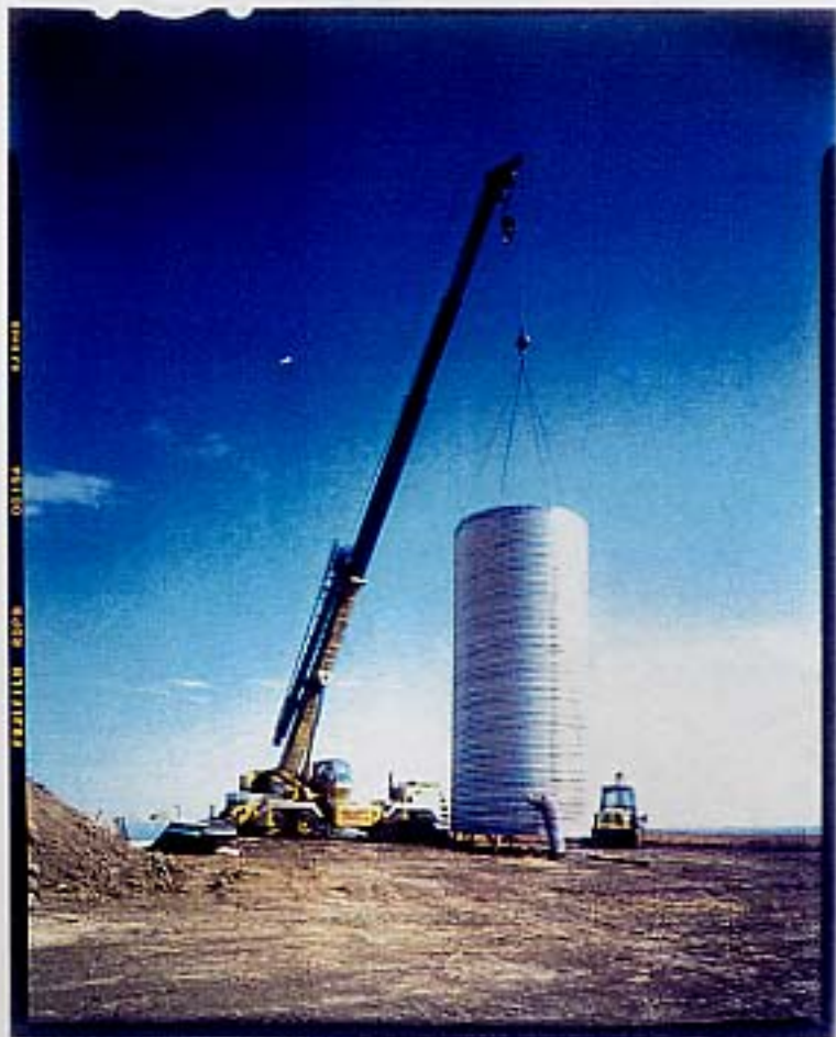
SET CMP IN EXCAVATION (VERTICAL)
