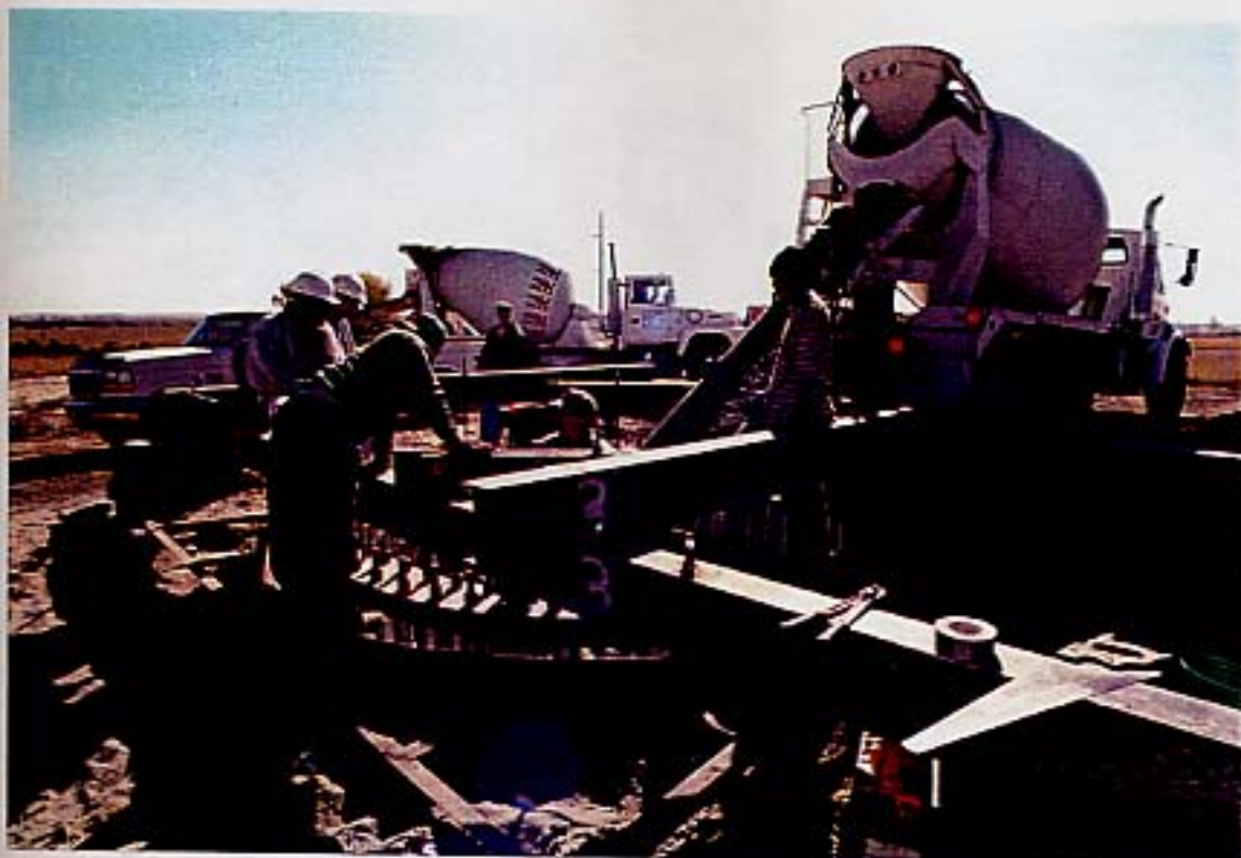
PLACING CONCRETE
