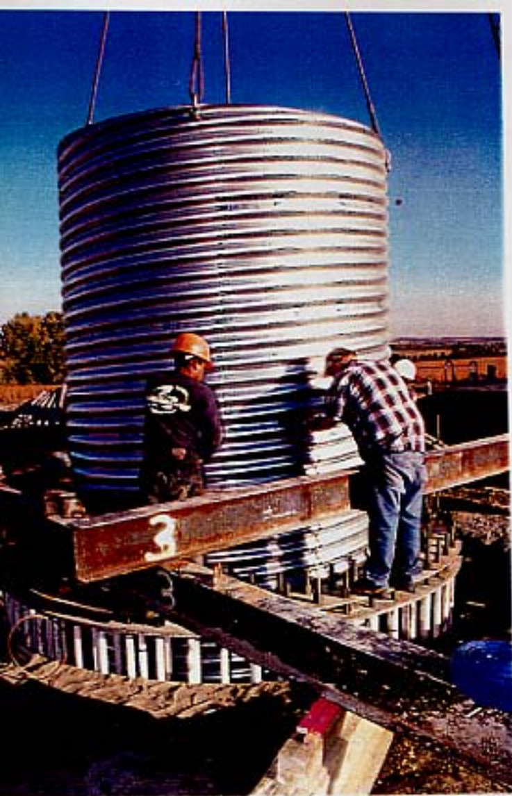
PLACING INNER CMP INSIDE ANCHOR BOLT
