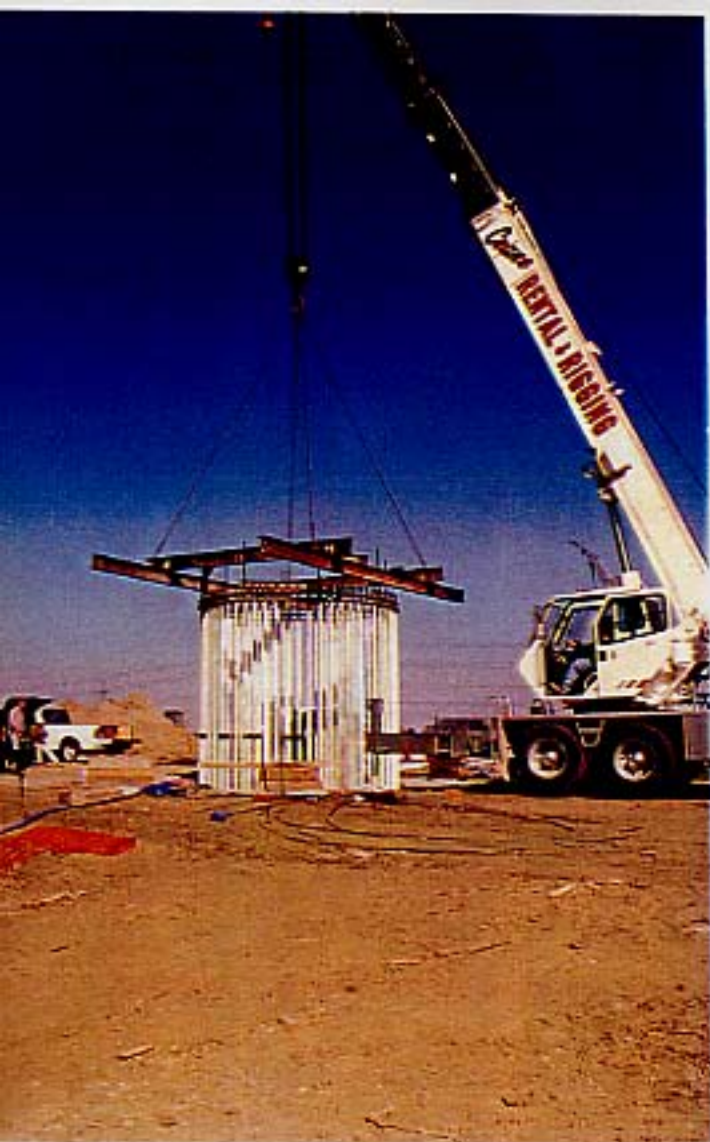
LIFTING ANCHOR BOLT CAGE TO INSTALL REBAR HOOPS
