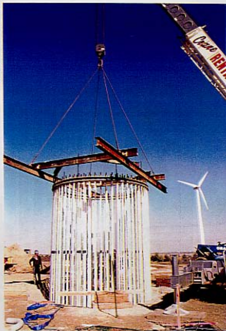
LIFTING ANCHOR BOLT CAGE
