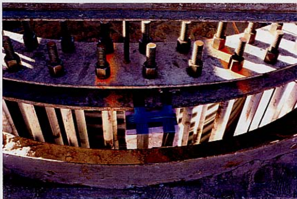
STYROFOAM BLOCKOUTS IN-PLACE
