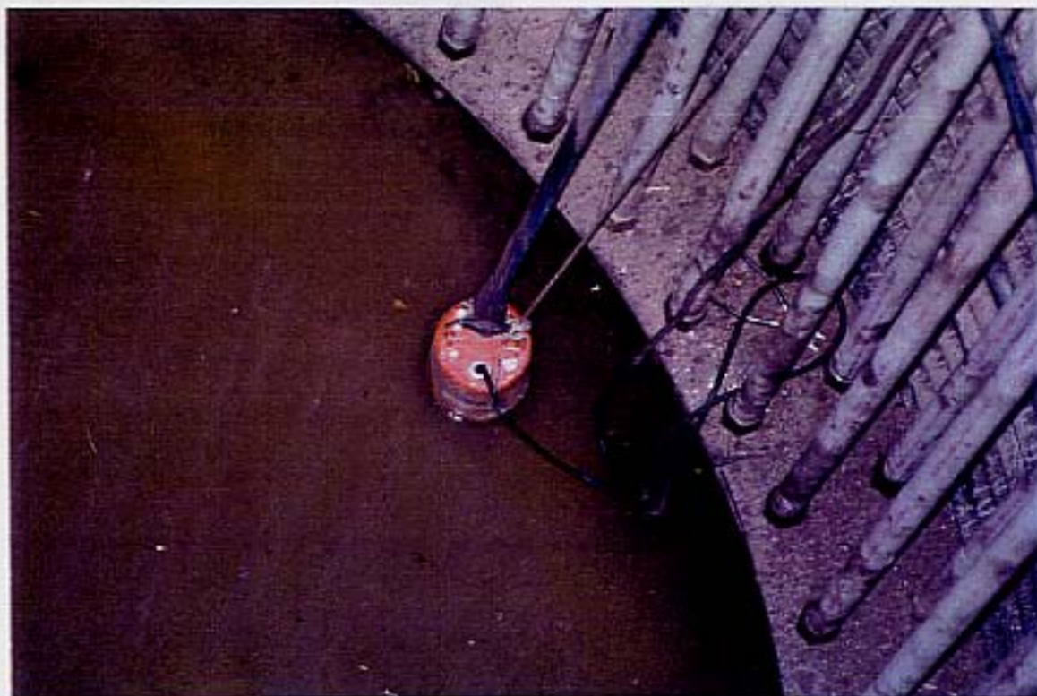
REMOVAL OF NUISANCE WATERS FROM BOTTOM OF EXCAVATION
