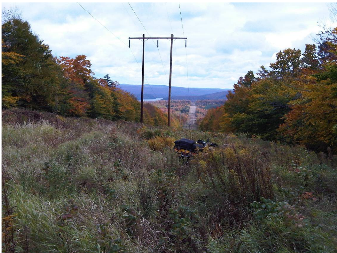
Photo 6: Mile 6 of existing transmission line viewed toward east.
