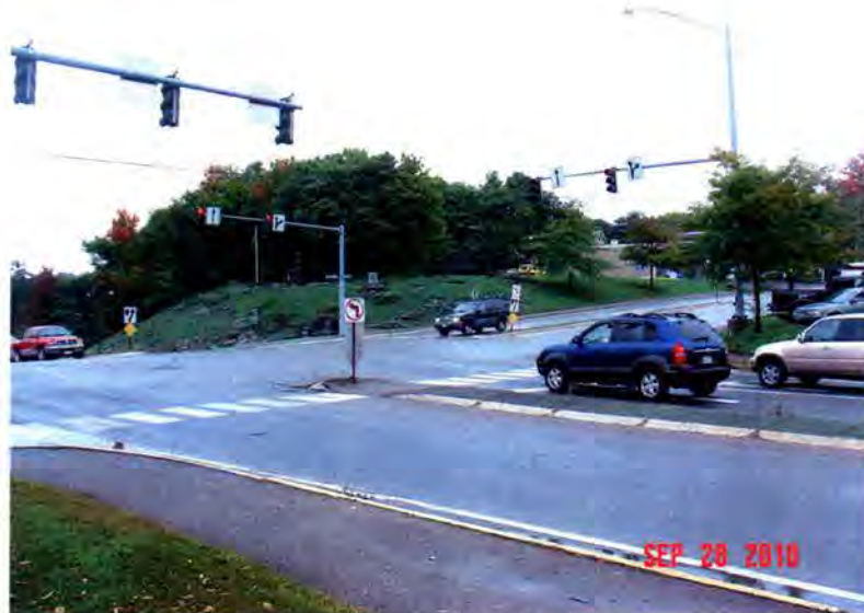
Intersection State Street & Route 9, Brewer, Maine
