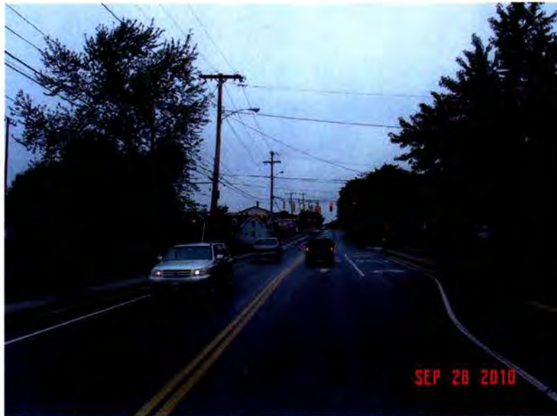
Signals at State Street & Eastern Avenue, Brewer, Maine
