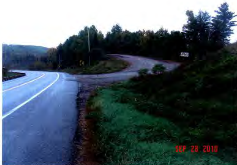
Entrance at Route 9 and 73-00-0 Road (Spectacle Pond Road), Aurora, Maine
