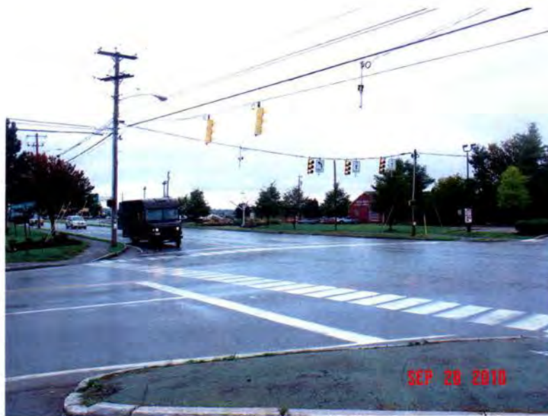
Intersection Parkway South & US 1A, Brewer, Maine
