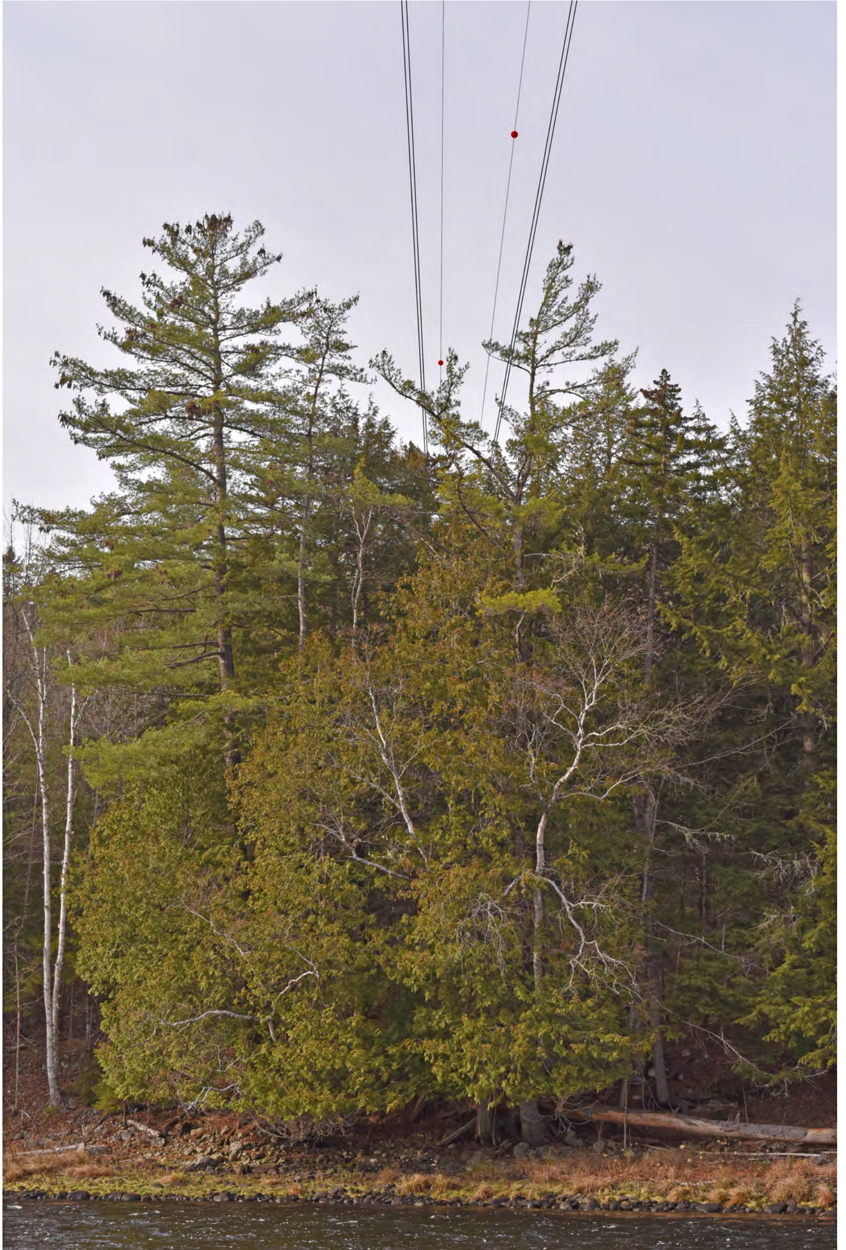
Proposed Conditions: Normal view looking northwest from the center line of the proposed HVDC transmission line crossing of the Kennebec River. The closest structure, screened by forested buffer in this view, would be 990' +/- to the northwest of this viewpoint.
