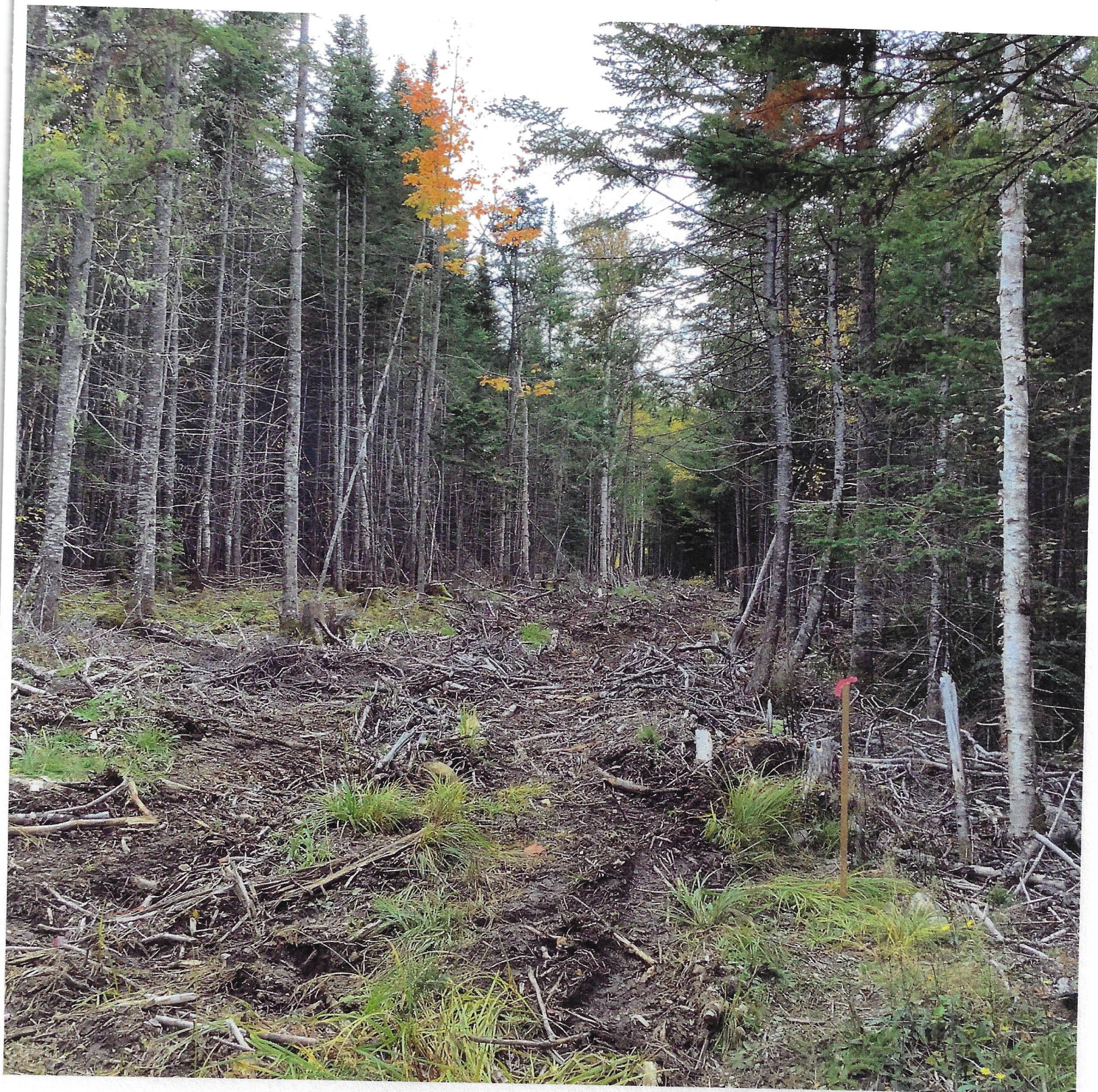
SKIPPED ROAD LOOKING WEST FROM 10/5/21 TOWER SITE TOWARDS SHALE PIT.
