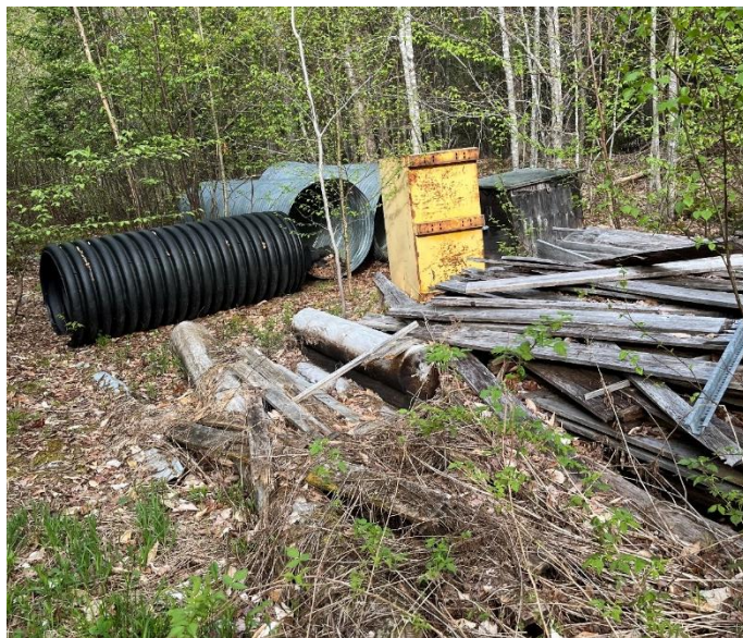
Figure 4: Remaining Materials on Site
