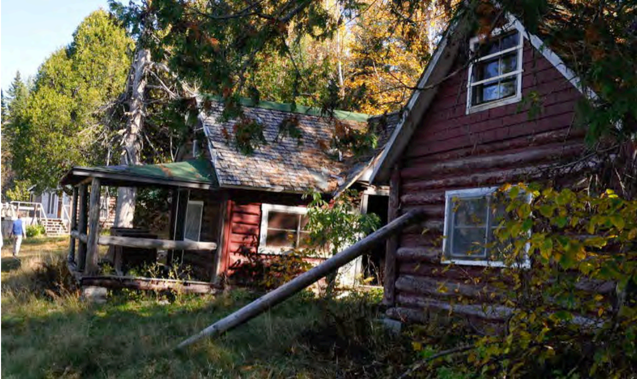
Two of the seven remaining cabins at the Yexas Camps
