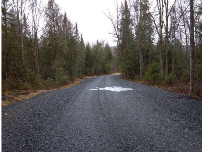
7. Example gravel road using crushed ripped ledge material near Long Lake.
