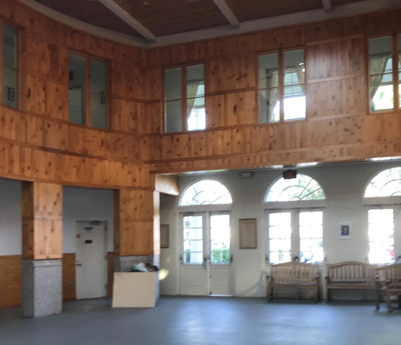
Maine Building First Floor Interior view, rotunda
