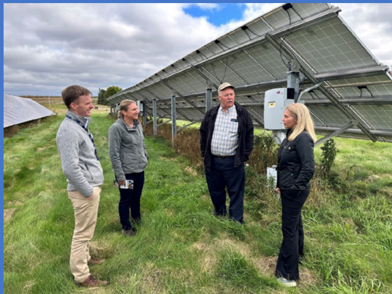
Limestone Solar Committee Chair Chuck Kelley explains to GOPIF staff the improvements to a newly purchased solar array that will power the town office and Maine School of Science and Mathematics. (Photo credit: Ryan McDonald, MSSM)
