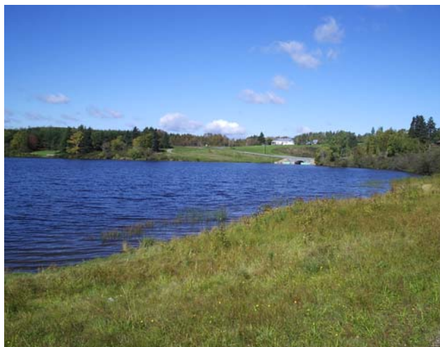
View from the east shore of the pond toward the outlet structure on the north end of Monson Pond.
