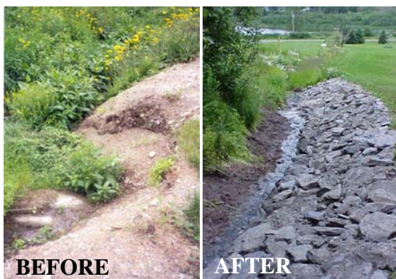
Stabilizing eroding waterways with stone rip-rap helps to prevent soil erosion.
