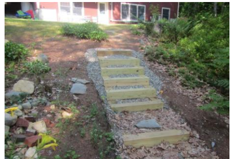
Example of infiltration steps installed by the BRCA YCC. (Source: BRCA)
