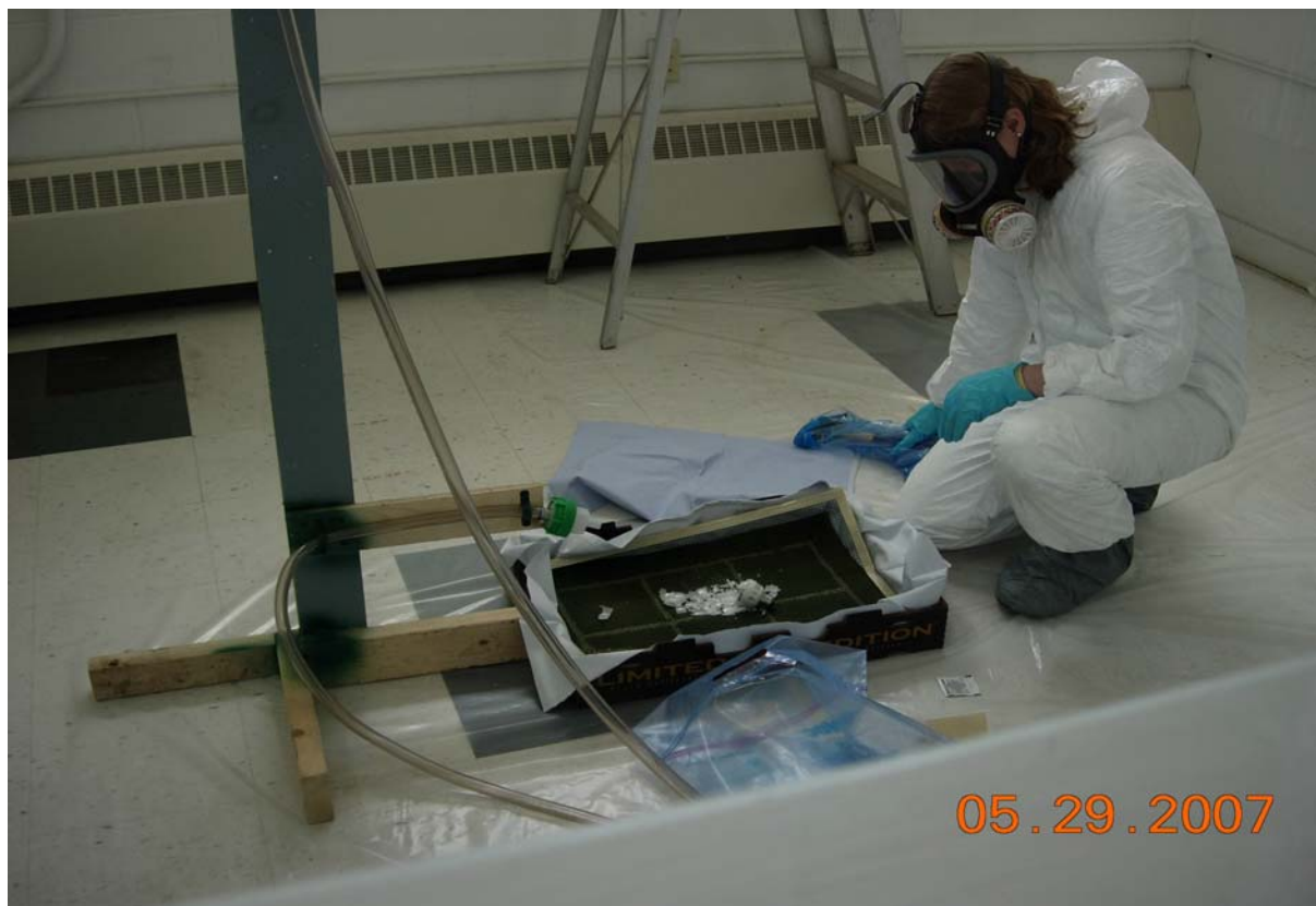
Figure 5-3. Thoroughly broken CFL
